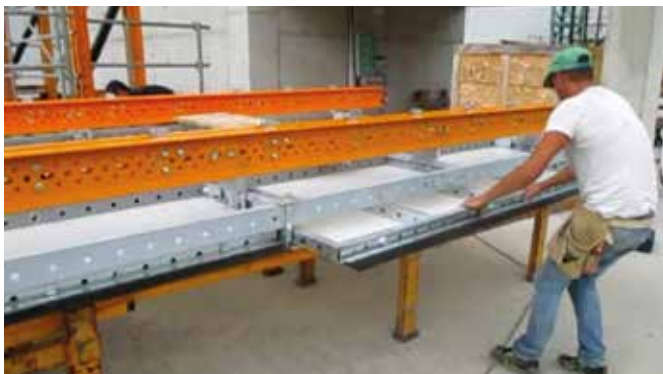
Manual sliding of telescopic panels for on-site placement
