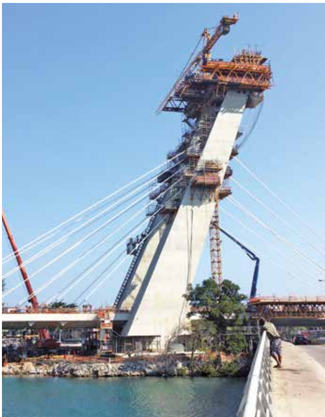
ATR used in inclined pylon construction
