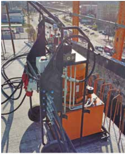
Self-climbing system, hydraulic power unit and cylinders
