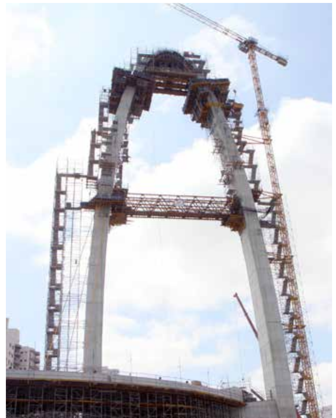
ATR used in inclined pylon construction
