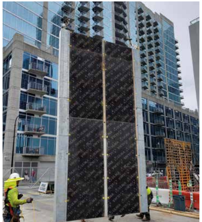
Lifting the gang of MEGALITE panels and STRIPPING CORNERS MAX
