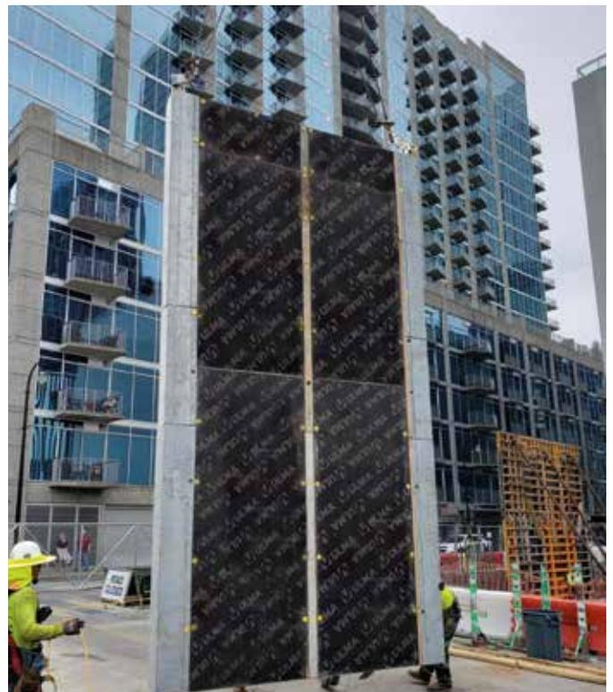
Lifting the gang of LGW panels and STRIPPING CORNERS MAX
