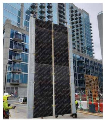
Lifting the gang of LGW panels and STRIPPING CORNERS MAX
