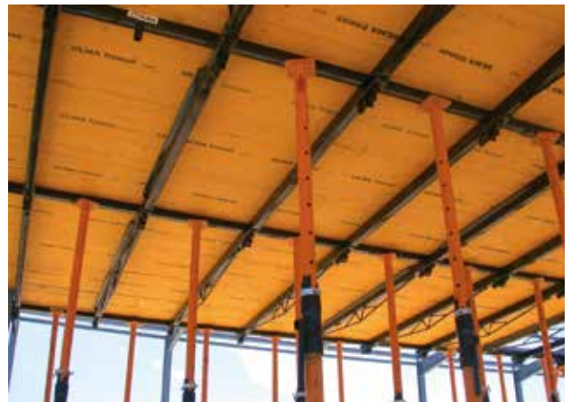
▲ 3-layer board Trimax in RAPID horizontal formwork ▲
