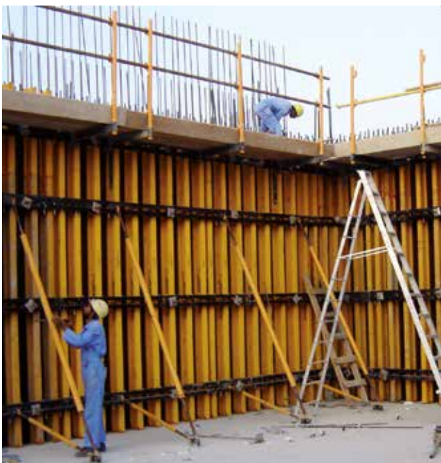
▲ VM-20 beams in ENKOFORM V-100 vertical formwork ▲
