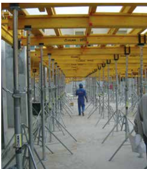
▲ VM-20 beams in ENKOFLEX horizontal formwork
