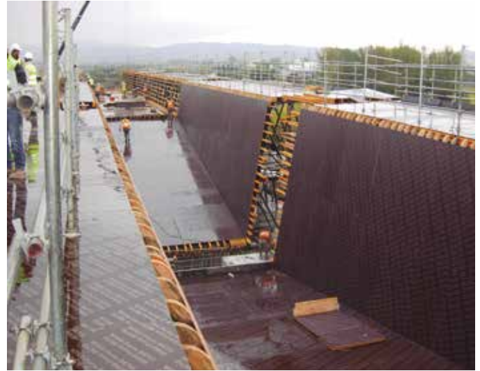
▲ Phenolic plywood as shuttering face in ENKOFORM H-120 formwork of a viaduct under construction
