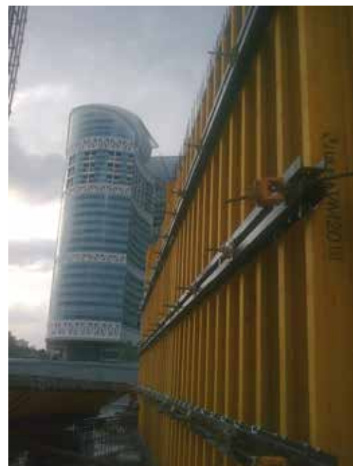
▲ VM-20 beams in ENKOFORM V-100 vertical formwork ▲
