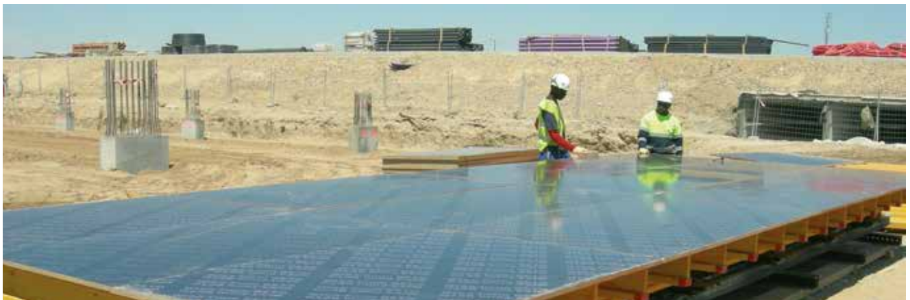
▲ Assembly of Table VR horizontal formwork with phenolic plywood and VM-20 timber beams
